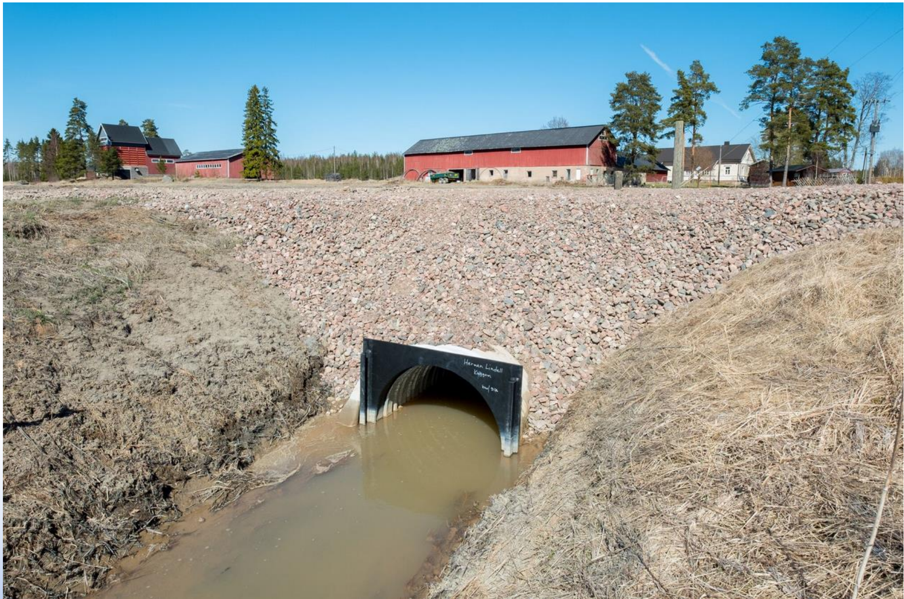
Constructions for control of the water levels at summertime
