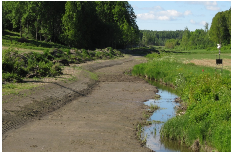
Ritobäcken, Sipoo (4 months after construction)
